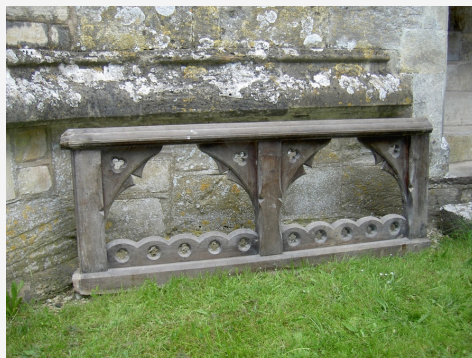
Picture 2. (Altar Rail) There are 2 similar rails though only 1 is shown. Approx. dimensions (for a single rail): Width 1610mm; Height 650mm
